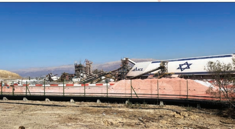
Dead Sea Works' main facility in Sodom, where potash, bromine, magnesium and salt are extracted from the water. The original company was founded in 1929. It now makes table salt, deicers and cosmetics, and is the world's 4th largest producer of potash.
